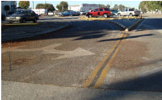
Reconfigure and upgrade main parking lot.
